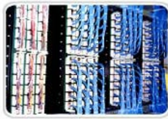
UTP patch panels in a rack
